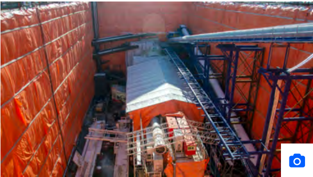
The Scarborough subway extension is taking shape. Here is a closer look
